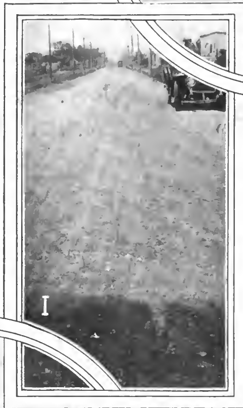
H—Another example of a road surface running parallel to that shown in Fig. G, but with a surface so soft that even a person's footprint makes an impression on the surface. The road shown on the right of the picture is being prepared for a tar surface
